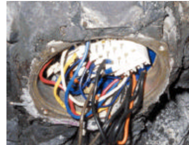
Post Fire Inspection
