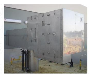
Incorporating high performance thermal insulation materials encapsulated by stainless steel skins, Darshield™ is supplied in pre-fabricated panel form for assembly and installation onsite or in the factory. Forming a rigid PFP enclosure, the panels are held together using bolts and captive nuts, with the final construction providing the necessary structural integrity to withstand the specified fire and blast conditions.
